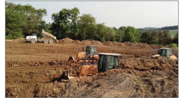
Photo 5 – Hauling and spreading topsoil before seeding.
